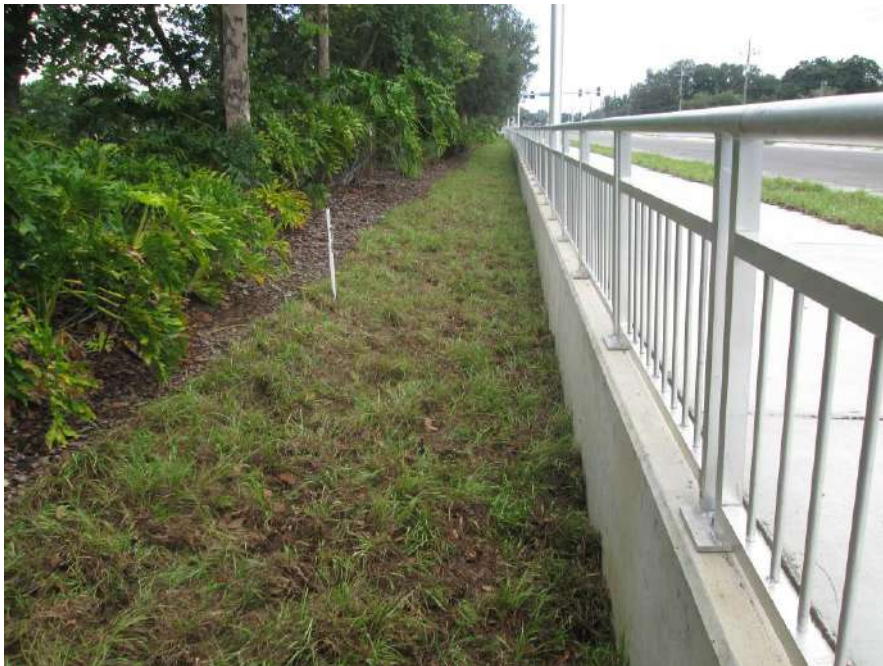
Viewing north from behind new railing south of Waterlefe Blvd
