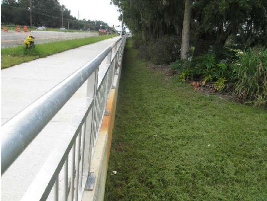
Viewing south from behind new railing north of Waterlefe Blvd
