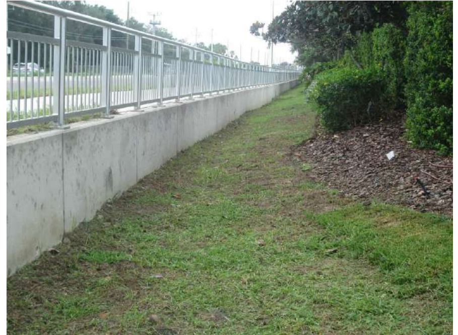
Viewing south from behind new railing south of Waterlefe Blvd
