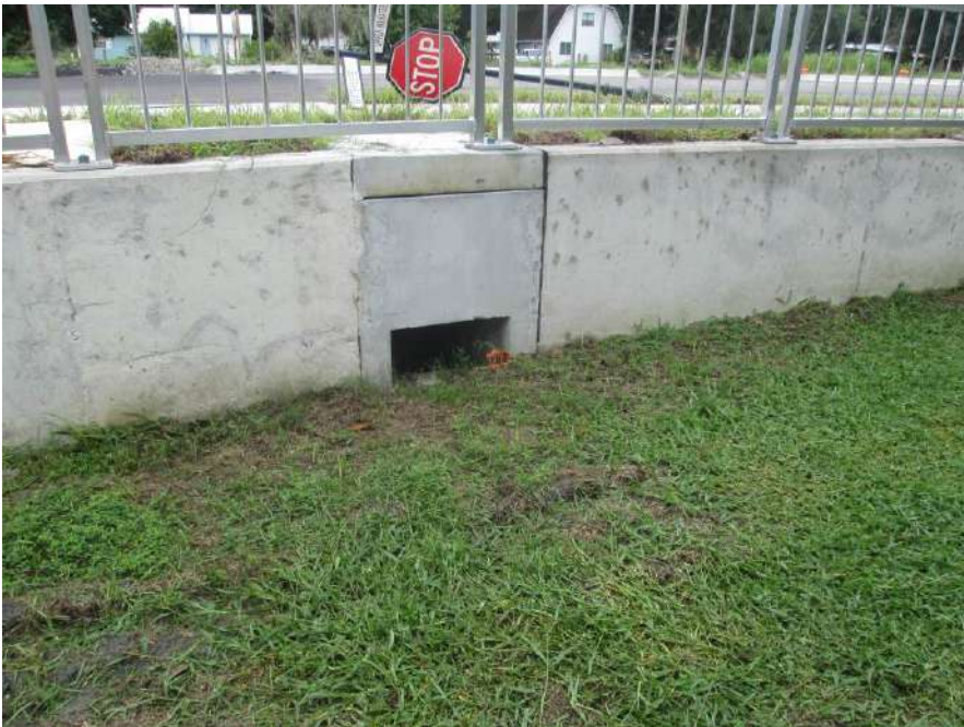
Drainage structure behind new sidewalk south of Waterlefe Blvd
