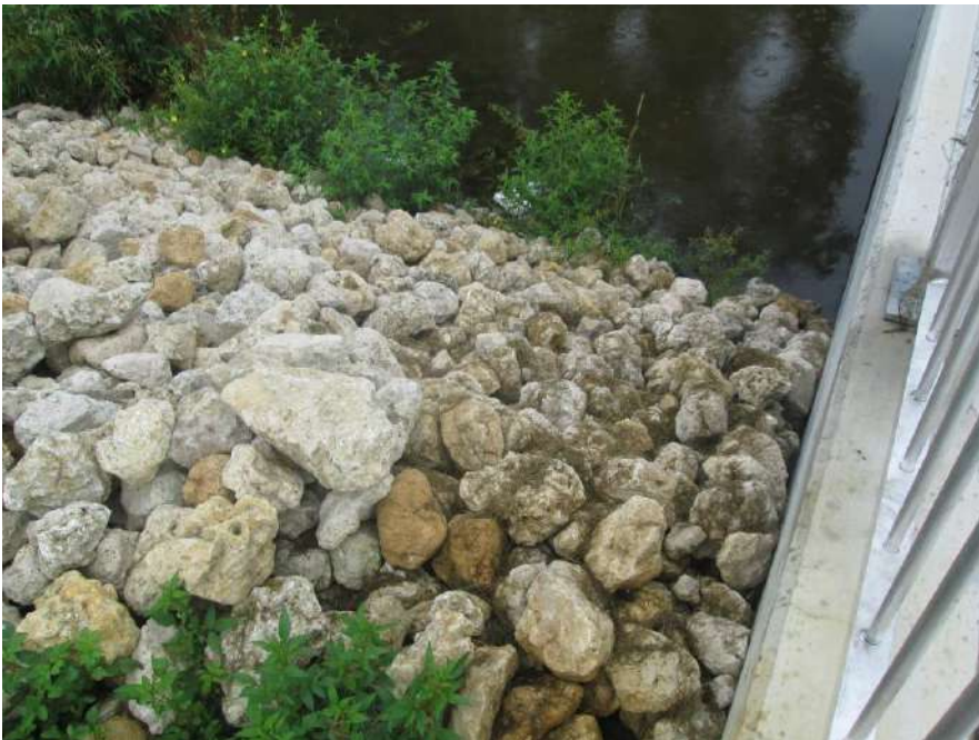
Rip rap on south side of channel that leads to Manatee River
