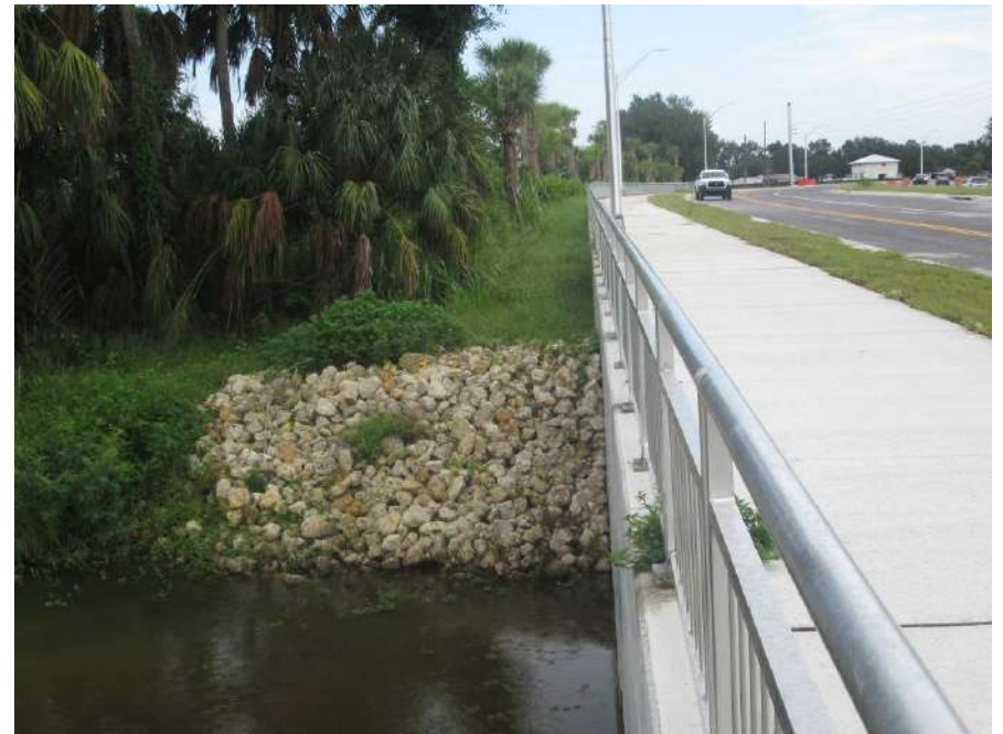
Rip rap on north side of channel that leads to Manatee River
